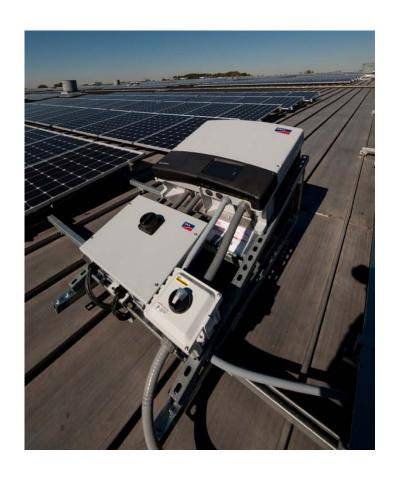
1MW commercial rooftop 42x STP 24000TL-US Shaw Industries Dalton, GA Installed by: Radiance Solar
